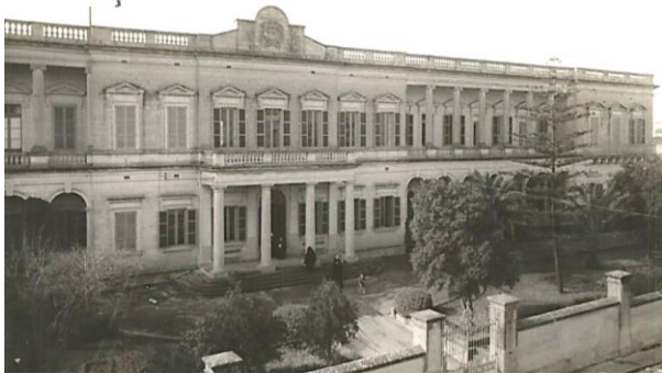
Front Façade (looking northeast)
